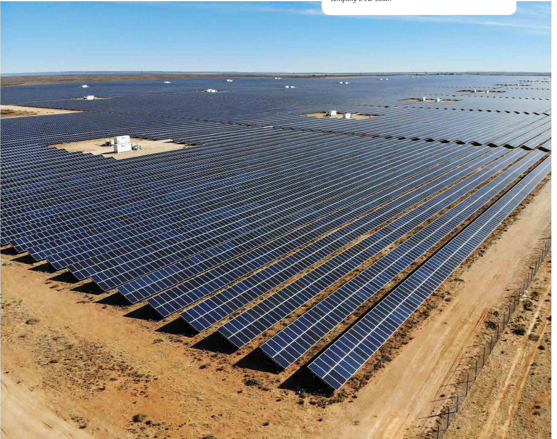
The solar PV plant at Prieska has a total of 275,760 polycrystalline panels, manufactured by Chinese company BYD Solar.
