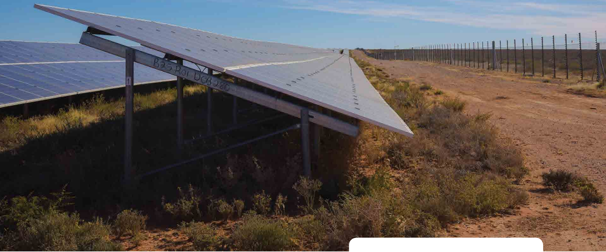
The solar PV plant at Prieska has a total of 275,760 polycrystalline panels, manufactured by Chinese company BYD Solar.
