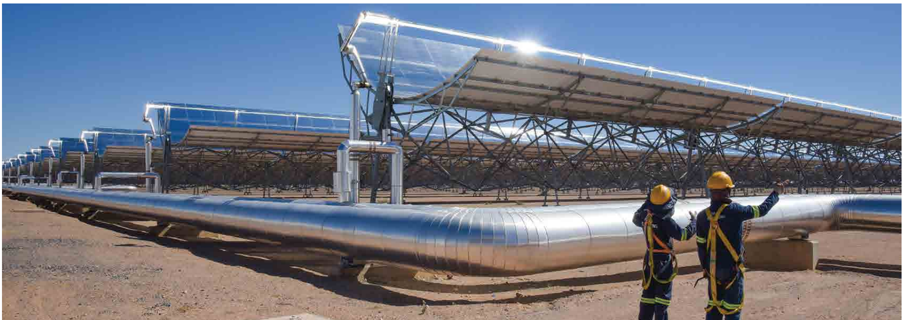
Glinting in the sun, the parabolic trough collectors tower above the the pipe carrying the heat transfer fluids, which gets increasingly wider the closer to the power block it gets.
