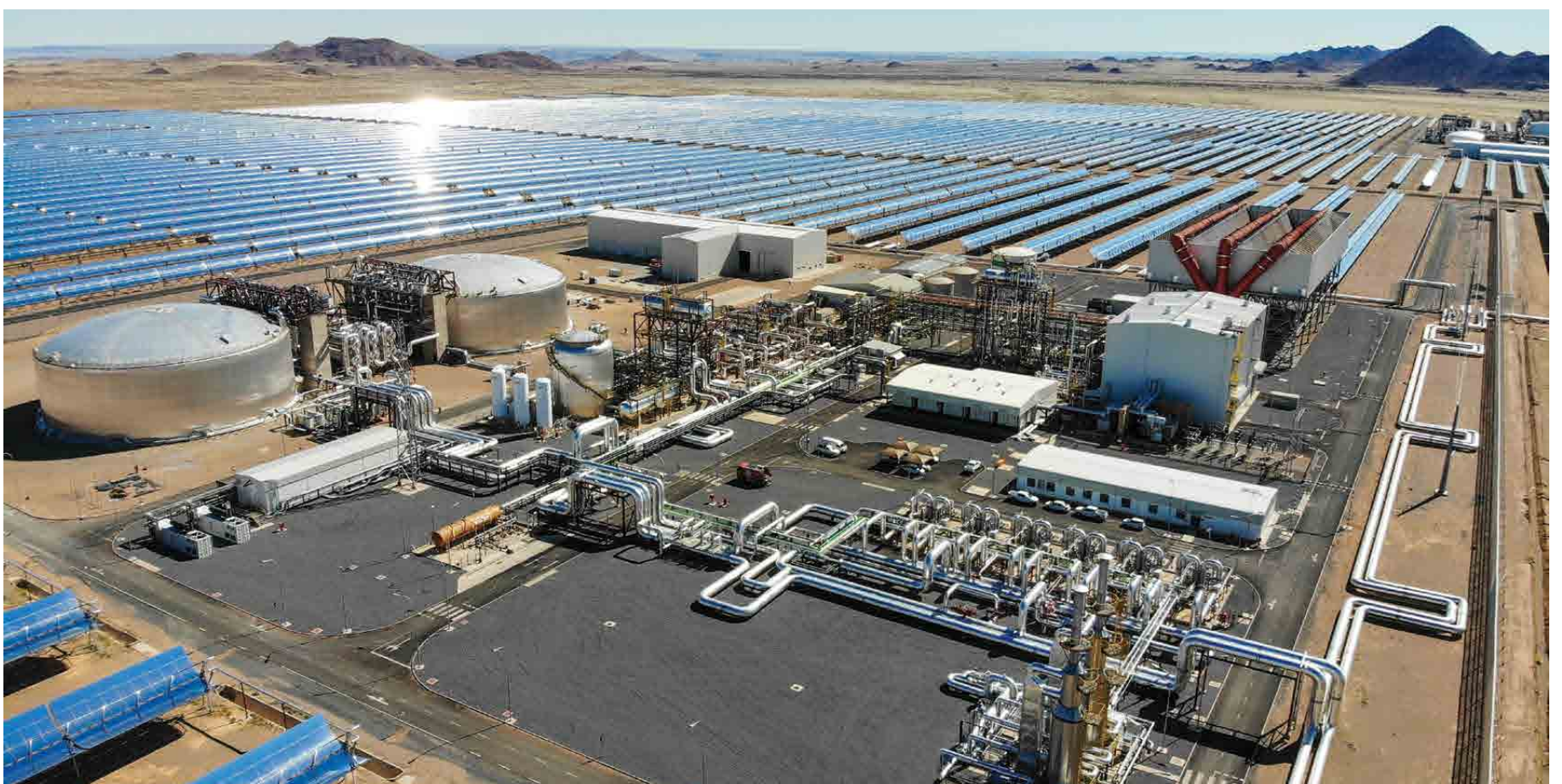
The power block sits in the centre of the rows of parabolic trough collectors.
